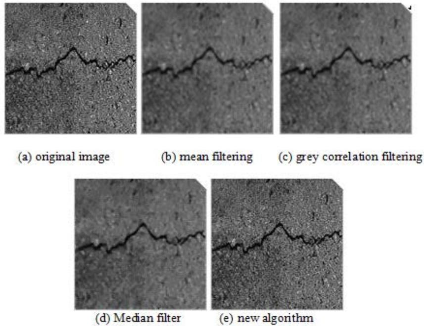
Fig. 4 algorithm results of the road surface image
