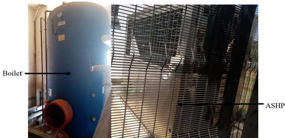
Figure 1. Installed ASHP and retrofitted electric boiler used in the study
