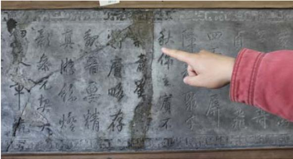
Figure 2. Cracks and brokenness of stone tablet.
