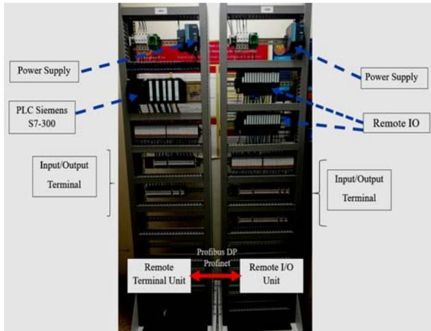
Figure 3. Main controller hardware.
